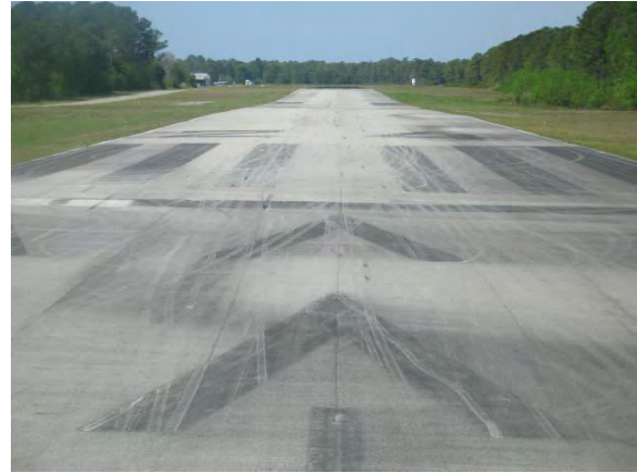
FIGURE 4-16. MARKINGS ARE OBSCURED BY ALGAE.
