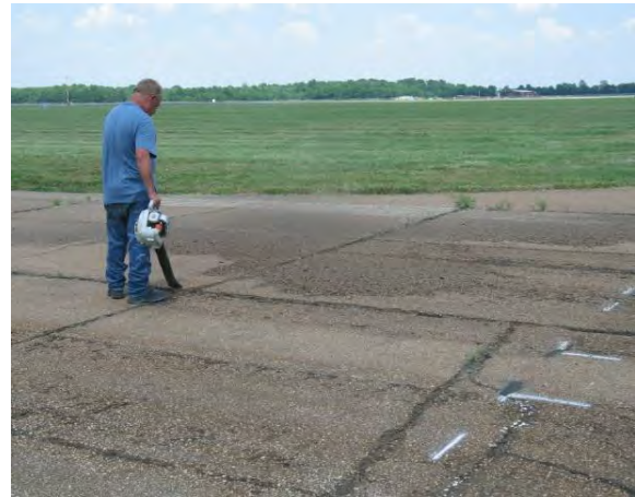
FIGURE 4-45. LEAF BLOWER CLEANS LOOSE RESIDUE AFTER SURFACE PREPARATION.
