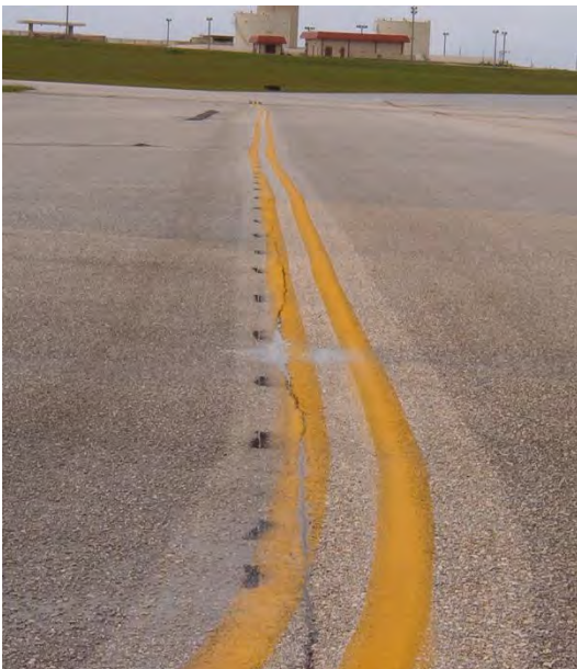
FIGURE 2-4. MARKING IS OUT OF ALIGNMENT
