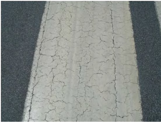
FIGURE 4-6. THIS MARKING IS 30 MONTHS OLD AND CRACKED.
