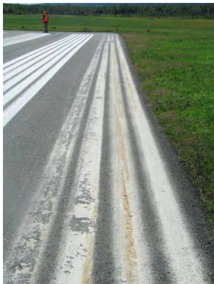
FIGURE 6-14. LAYERED STRIATIONS ON THE SIDELINE WERE SCRAPED OFF BY SNOWPLOWS.
