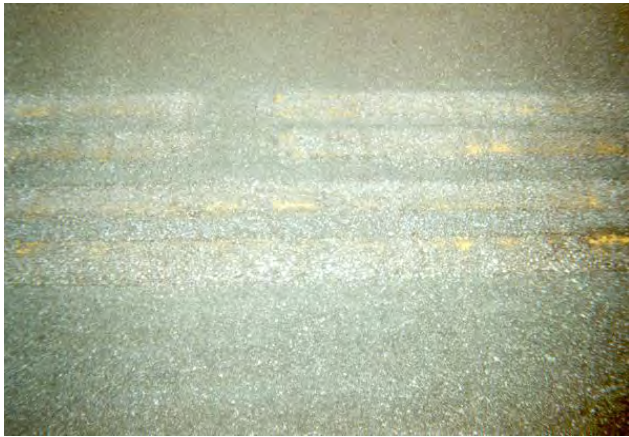
FIGURE 5-8. MINIMAL GRINDER SCARS ON ASPHALT AFTER REMOVING 90 PERCENT.
