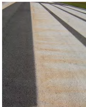
FIGURE 4-26. STAINED LEADING EDGE OF MARKING FROM IRON CONTAMINANTS.
