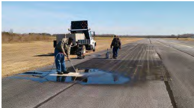
FIGURE 4-42 – PRESSURE WASHER, BY HAND.
