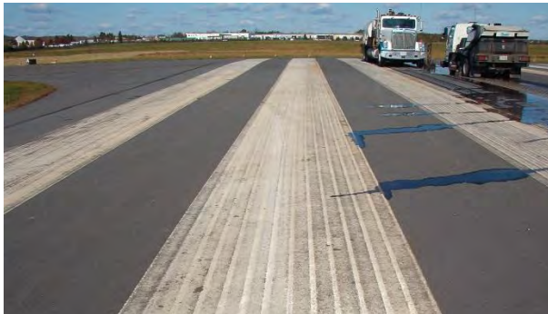
FIGURE 4-1. BEFORE CLEANING LOOSE AND POORLY BONDED PAINT.
