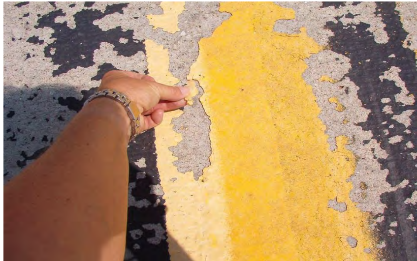
FIGURE 4-49. LOOSE PAINT FOUND AFTER SURFACE PREPARATION. PAINT REMOVAL WAS NEEDED. 7
