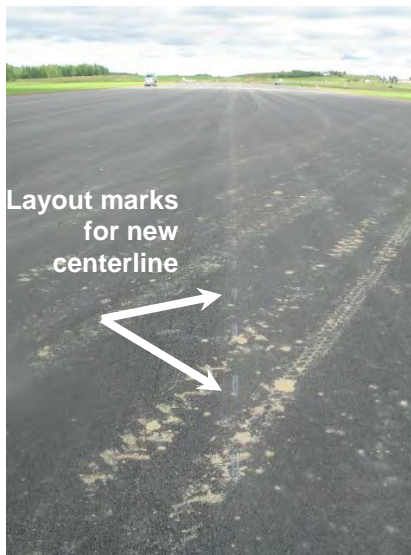
FIGURE 6-2. CONSTRUCTION DIRT MUST BE CLEANED.
