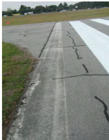
FIGURE 4-17. WATER FROM THE AIRPORT'S FIRE TRUCK, WITH 150 PSI, RINSED THE SIDELINE.
