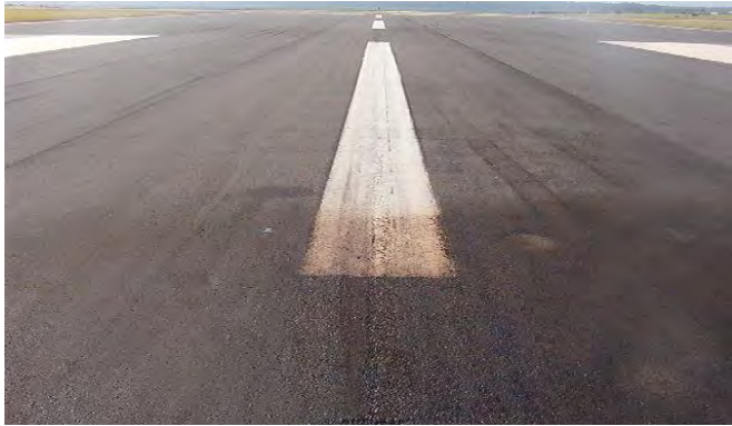
FIGURE 4-36. THE OILY STAIN WILL PREVENT NEW COATING FROM BONDING.
