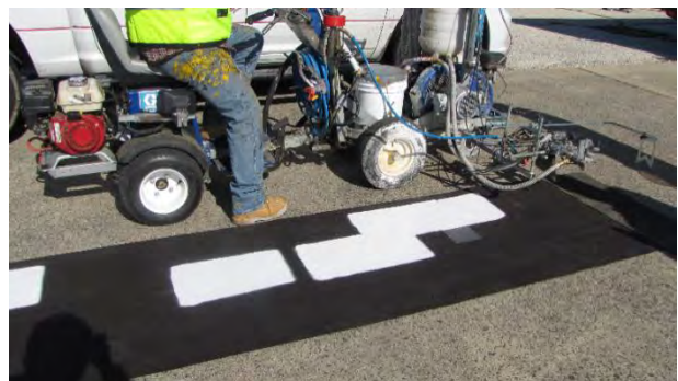
FIGURE 6-58 TEST LINES ON TAR PAPER.
