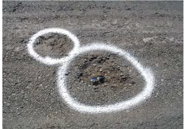
FIGURE 5-24. PRE-EXISTING CONDITION CAUSED BY OIL SPILL THAT SOFTENED THE ASPHALT.
