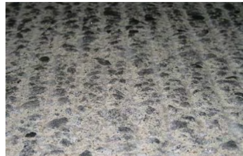
FIGURE 5-17. AFTER TEN YEARS OF SHOTBLASTING TO REMOVE RUBBER DEPOSITS.
