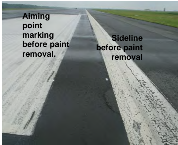
FIGURE 5-27. BEFORE PAINT REMOVAL. FIGURE 5-28. AFTER PAINT REMOVAL.
