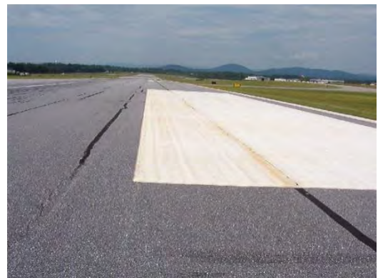
FIGURE 6-11. JOINT MATERIAL DISCOLORS THE WHITE PAINT.
