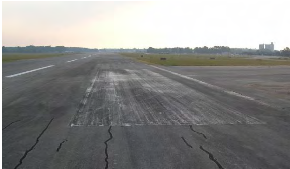
FIGURE 4-19. BEFORE WATERBLASTING: ALGAE OBSCURE MARKING.
