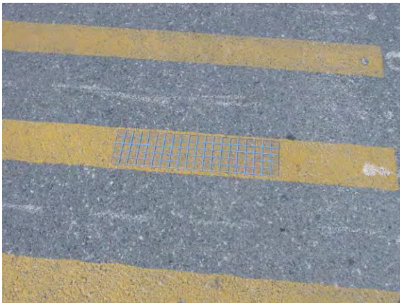
FIGURE 2. A 5- x 20-inch grid for a six-inch line.
