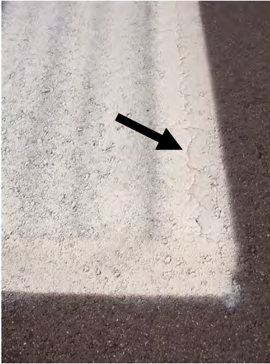
FIGURE 4-14. PAINT CRACKS WHEN APPLIED TOO THICKLY.
