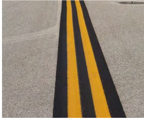
FIGURE 6-43. AIRLESS LINES HAVE SHARPER EDGES.
