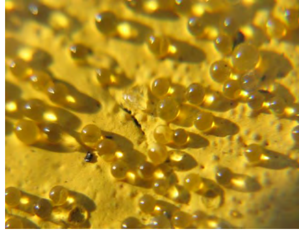
FIGURE 3-10. POOR TYPE IV BEAD EMBEDMENT.
