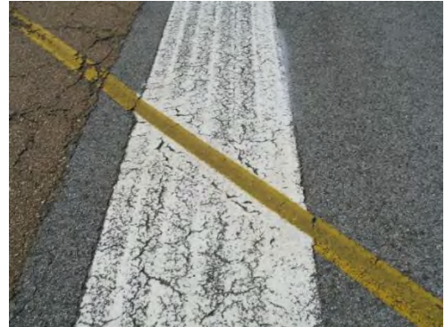
FIGURE 5-3. CRACKED AND PEELING MARKINGS –
