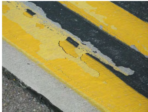
FIGURE 2-1. PEELING PAINT LAYERS
