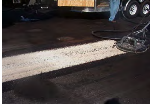
FIGURE 4-38. THE PROCESS USED TO REMOVE OIL STAIN.
