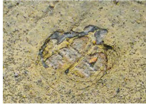
FIGURE 6-7. MULTIPLE LAYERS OF PAINT FILL THE GROOVES.
