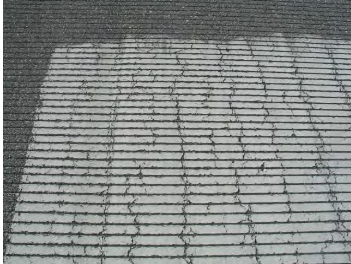
FIGURE 4-15. PAINT BONDS BETTER TO ASPHALT THAN ASPHALT DOES TO ITSELF.
