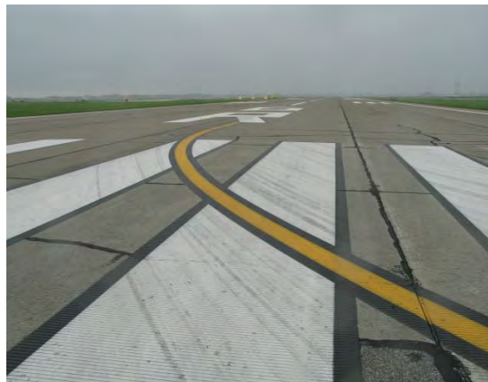
Twelve-inch taxiway centerline is painted over runway markings when it designates a SMGCS route.
