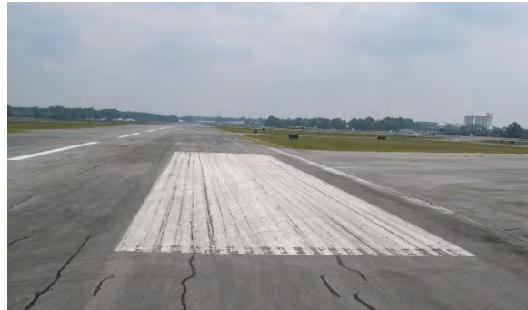
FIGURE 4-20. AFTER WATERBLASTING, BUT BEFORE PAINTING.
