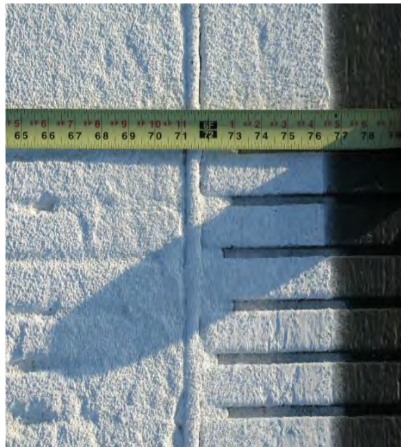
FIGURE 2-3. MARKING DIMENSION IS OUT OF TOLERANCE.
