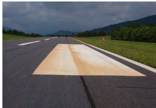
FIGURE 4-27. STAINED LEADING EDGE AND LOW AREA ALONG JOINT WHERE WATER FLOWS.
