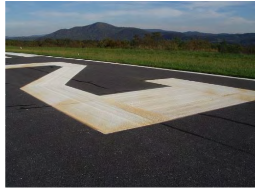
FIGURE 4-33. REPAINTING WITHOUT CLEANING THE STAIN RESULTS IN BLEED-THROUGH.
