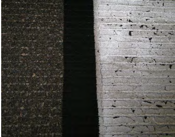
FIGURE 5-10. BEFORE PAINT REMOVAL.
