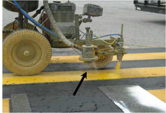
FIGURE 6-41. GLASS BEAD DISPENSER ON AN ATOMIZED HAND MACHINE.
