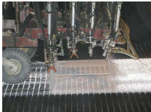
FIGURE 6-19. AIRLESS PAINT GUNS AND BEAD GUNS APPLYING MATERIAL TO PAVEMENT.
