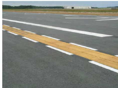
FIGURE 4-30. AFTER THREE YEARS USING STAIN RESISTANT FORMULA
