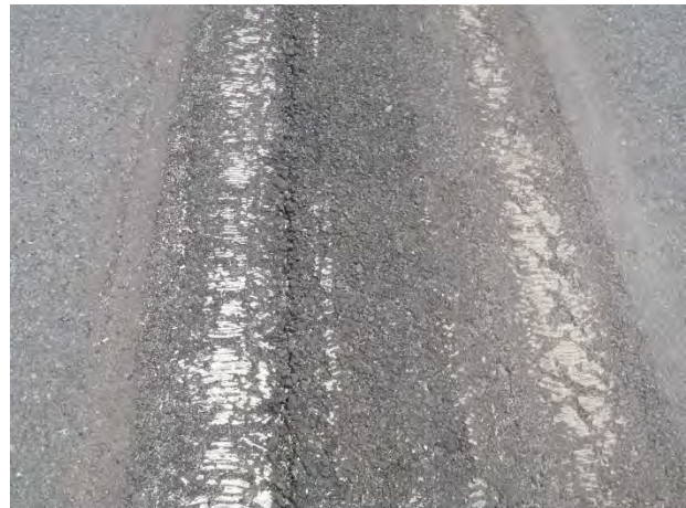
FIGURE 5-30. REMOVAL OF MULTIPLE LAYERS ON DETERIORATED ASPHALT.
