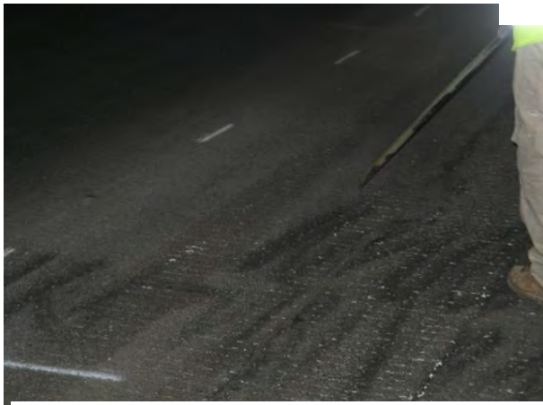
FIGURE 4-41. COMPRESSED AIR REMOVES FINE RESIDUE AFTER PAINT REMOVAL OPERATION.
