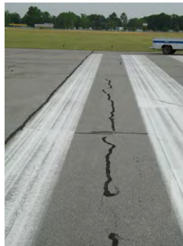
FIGURE 4-18. THE SAME SIDELINE AND THRESHOLD MARKING EIGHTEEN MONTHS LATER.
