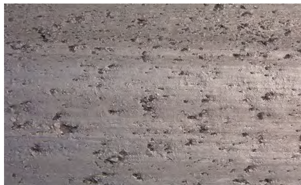
FIGURE 4-12. BEFORE RUBBER REMOVAL.
