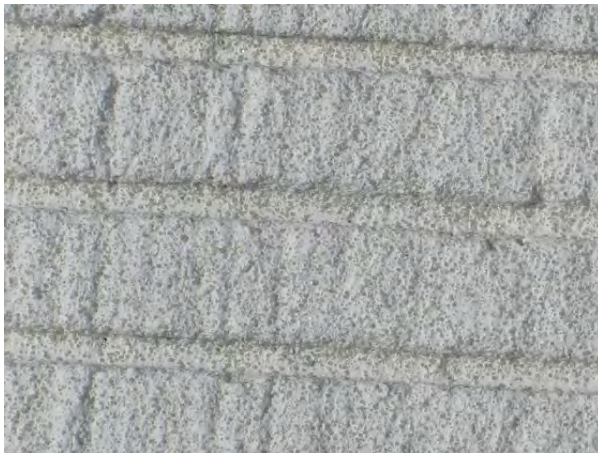
FIGURE 6-5. THE UNPAINTED SIDE OF THE GROOVES IS NOT NOTICEABLE FROM A DISTANCE.
