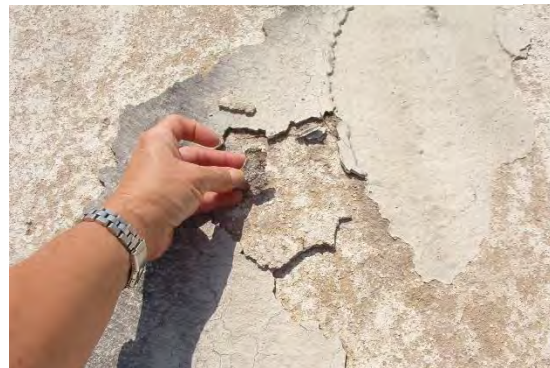
FIGURE 5-6. HEAVY PAINT BUILD UP ON CONCRETE.
