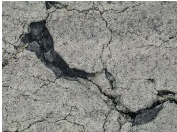
FIGURE 5-29. CRACKED PAINT INDICATES PRE-EXISTING PAVEMENT DETERIORATION.
