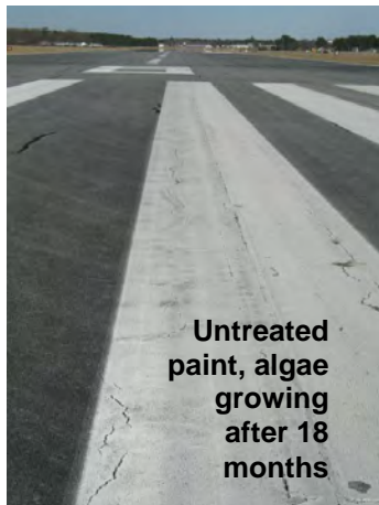
FIGURE 4-21. PAINT USED WAS STANDARD TT-P-1952E.
