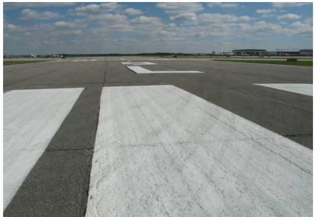
FIGURE 6-38. THE SAME MARKING AS IN FIGURE 6-37 DURING DAYLIGHT.
