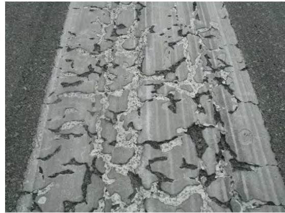
FIGURE 4-7. MANY LAYERS OF PAINT ON ASPHALT.
