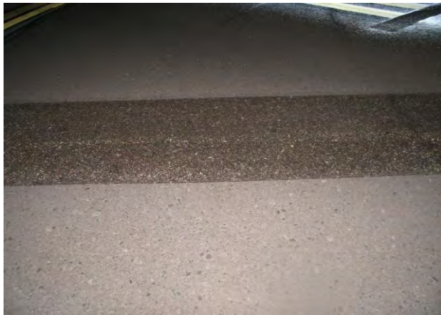
FIGURE 5-20. A SCAR FROM ULTRA-HIGH-PRESSURE WATERBLASTING ON GOOD ASPHALT.
