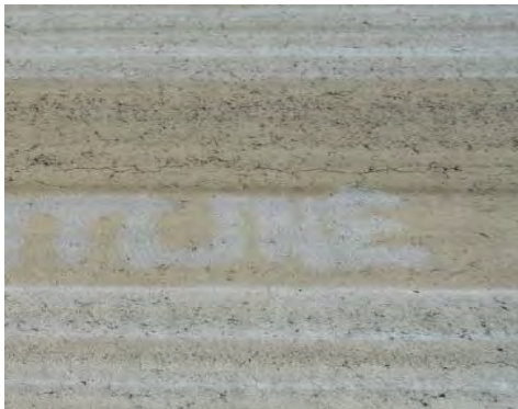
FIGURE 4-34. RUST REMOVER WHITENS STAINED MARKING WHERE “TLINE” WAS PRINTED.
