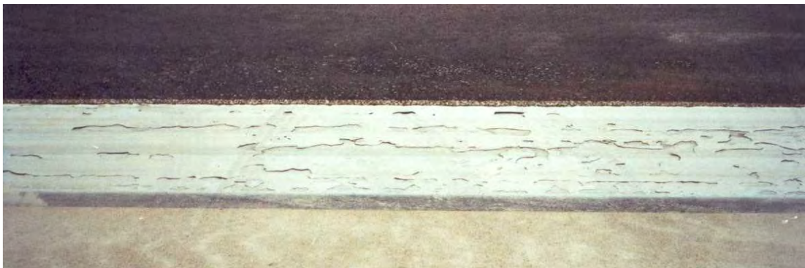
FIGURE 4-3. REPEATED PAINTING ON CONCRETE LEADS TO FOD.
