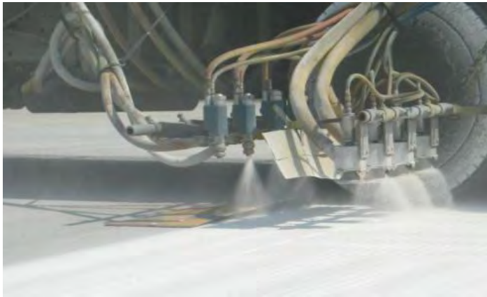
FIGURE 6-28. FOUR PNEUMATIC (ATOMIZED) PAINT GUNS APPLYING A 3-FOOT WIDE PATTERN.
