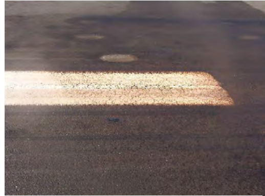
FIGURE 4-37. ANOTHER VIEW OF THE OIL-STAINED MARKING IN FIGURE 4-36.
