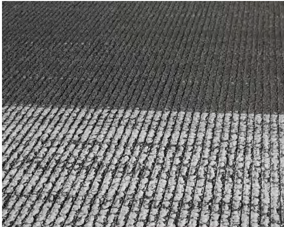
FIGURE 4-4. REPEATED PAINTING ON ASPHALT RESULTS IN PAINT BUILD UP, AND CRACKING OF PAINT AND PAVEMENT.
