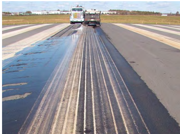
FIGURE 5-18. HIGH-PRESSURE WATER BLASTING IS EFFECTIVE FOR REMOVING PAINT ON SOUND ASPHALT SURFACES AS WELL AS ON CONCRETE.
