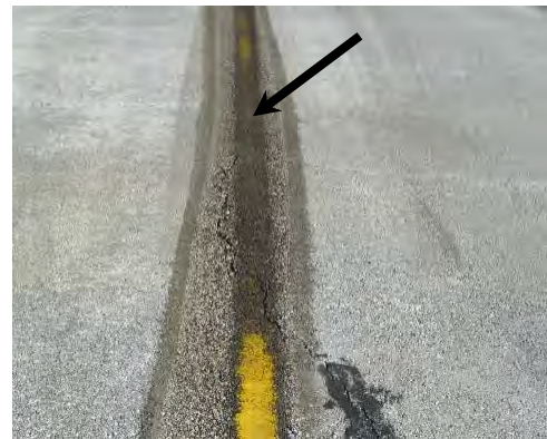
FIGURE 5-26. THE SCAR IS THE DARK PORTION OF THE ASPHALT THAT WAS SHIELDED FROM UV.
