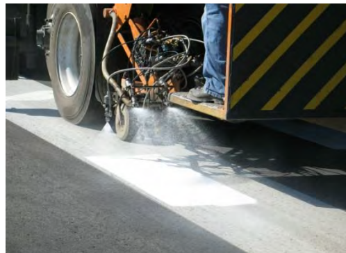
FIGURE 6-47. GLASS BEAD DISPENSERS ADJUSTED TOO HIGH.
