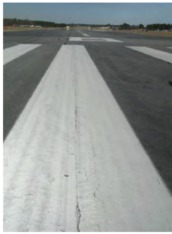
FIGURE 4-22. PAINT FORMULATED TO RESIST ALGAE.
