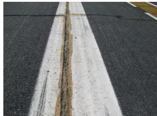
FIGURE 4-32. CENTERLINE IN FIGURE 4-31 THAT HAD CRACK SEAL AND “TOUCH UP” PAINT APPLIED.
