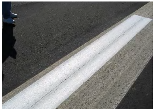
FIGURE 6-46. UNEVEN MATERIAL DISTRIBUTION, LIGHT ON THE EDGES OF EACH PAINT GUN.
