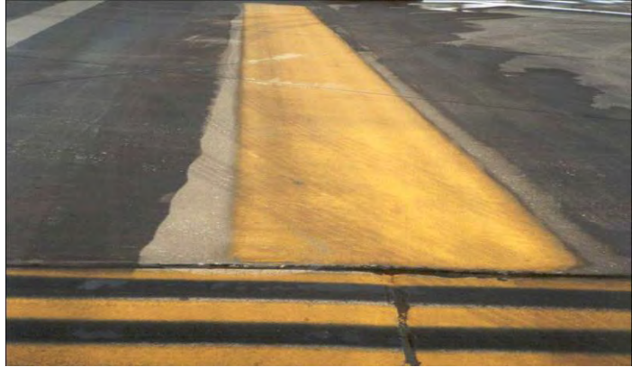
FIGURE 4-40. TAXIWAY SHOULDER MARKING WAS CONTAMINATED WITH OILY JET BLAST.
