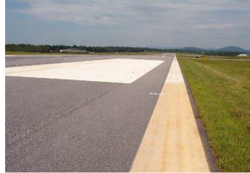
FIGURE 4-28. GROOVED SURFACE MAKES STAIN LESS NOTICEABLE.
