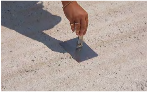
FIGURE 6-66. WET FILM GAUGE ON A METAL COUPON.
