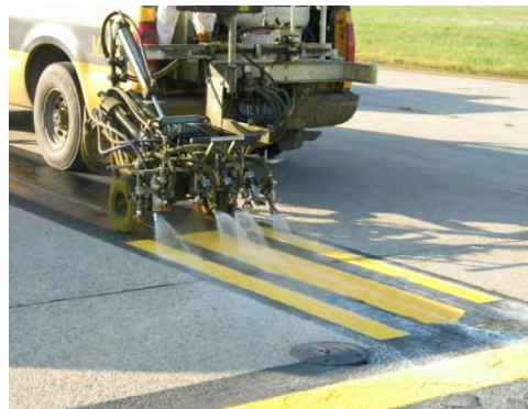
FIGURE 6-23. THREE PAINT GUNS AND FOUR BEAD GUNS APPLIED THE YELLOW PATTERN IN ONE PASS.
